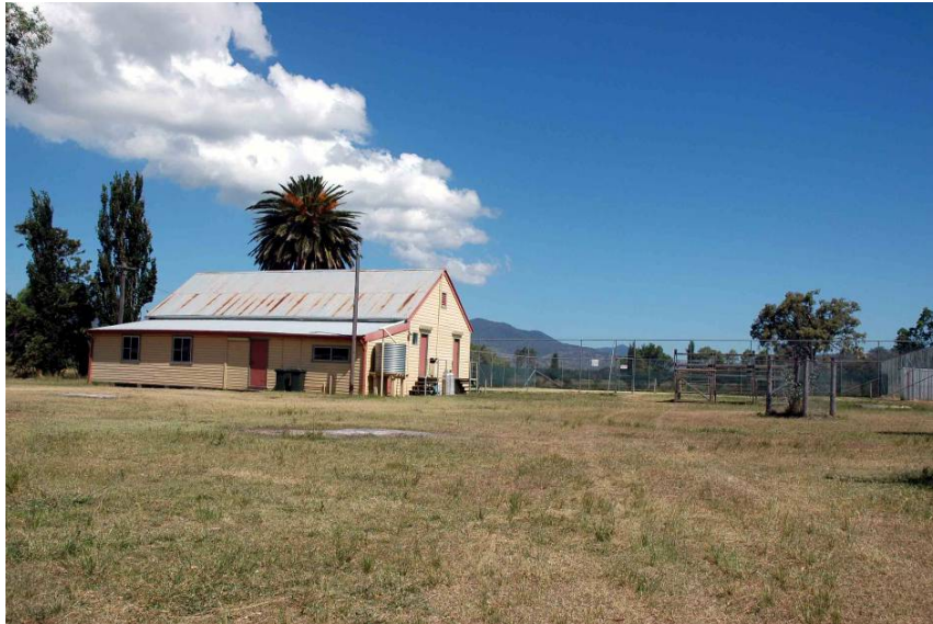
Photo 2.14: Warrah Creek Hall
