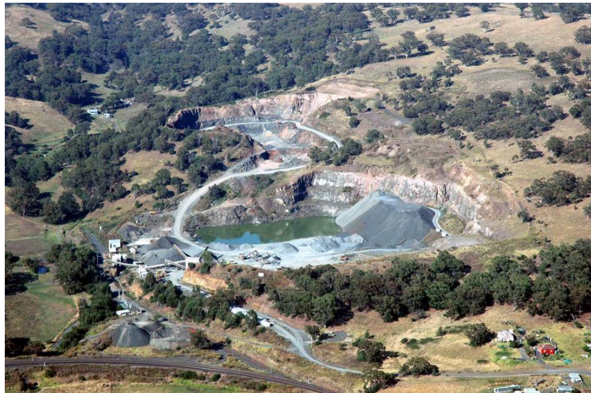
Photo 2.12: Ardglen Hard Rock Quarry
