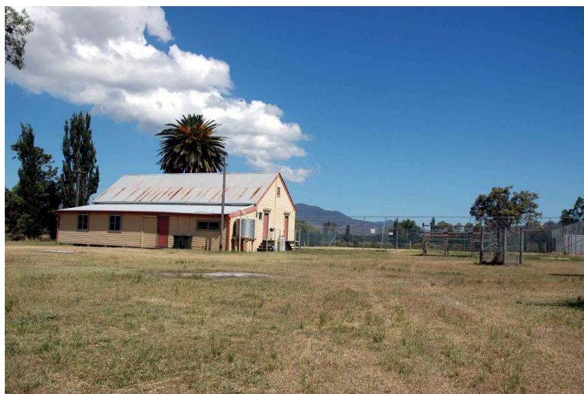
Photo 2.14: Warrah Creek Hall
